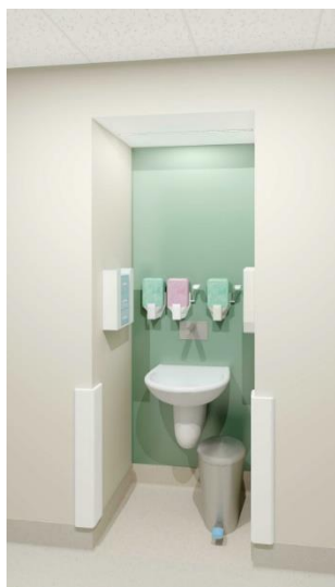
Figure 1.10: Reduced height ceiling within a hand wash bay along a corridor
