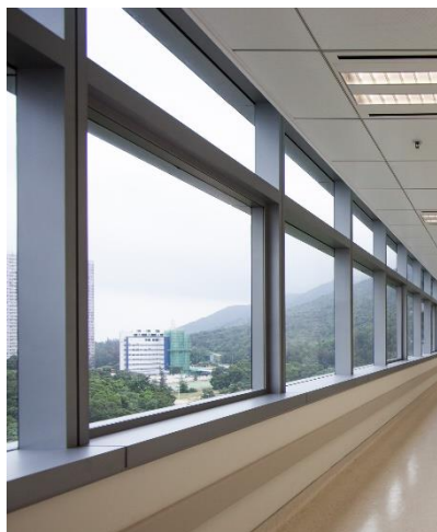
Figure 7.2: Fixed windows in corridor
