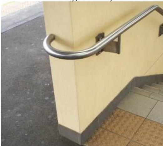
**Figure 6.5: Stair hand rail with return to the wall**
