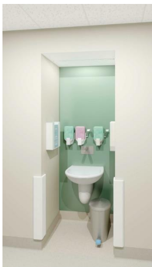
Figure 1.9: Reduced height ceiling within a corridor bay
