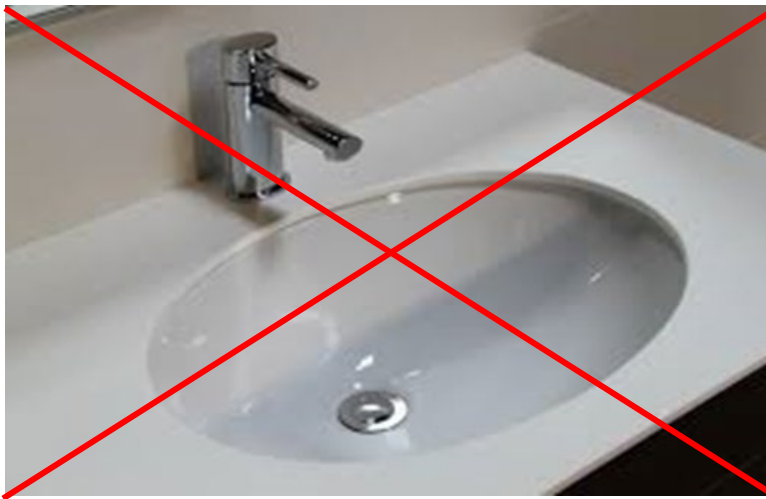
Figure 4: Under mount hand basin is not recommended
