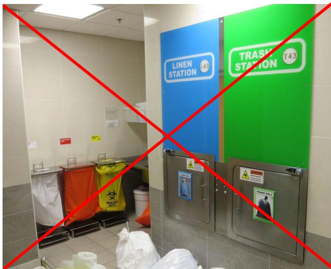
Figure 16: Linen and Waste chutes are not recommended
