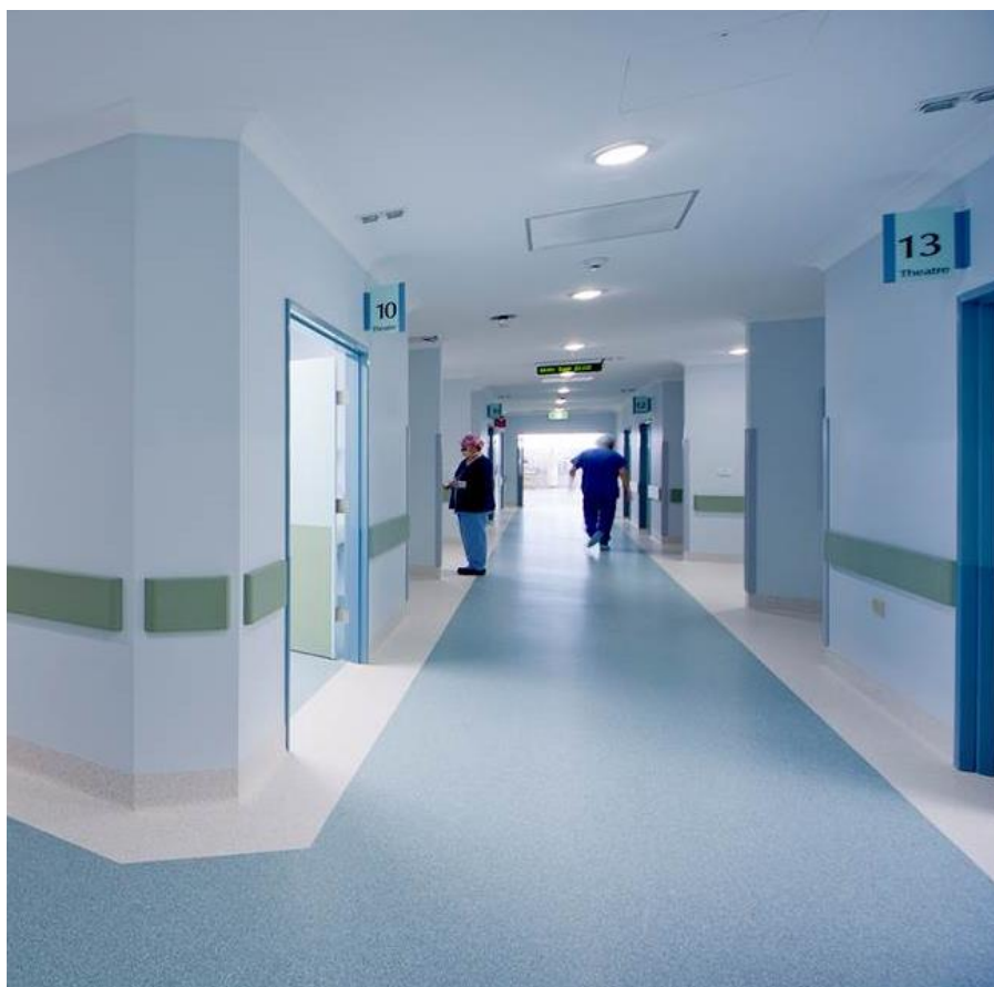
Figure 28: Floors and skirtings in clinical areas such as Operating Unit are integral and covered.
