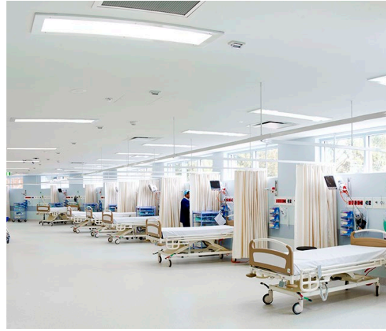
Figure 23: Monolithic ceilings in Stage 1 recovery areas
