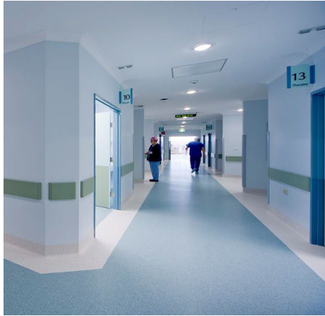
Figure 27: Floors and skirtings in clinical areas such as Operating Unit are integral and covered.
