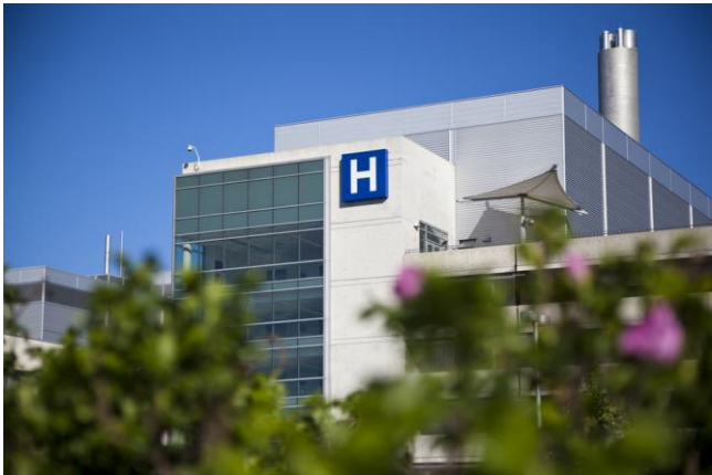
Figure 2: Hospital sign replicated on the building exterior
